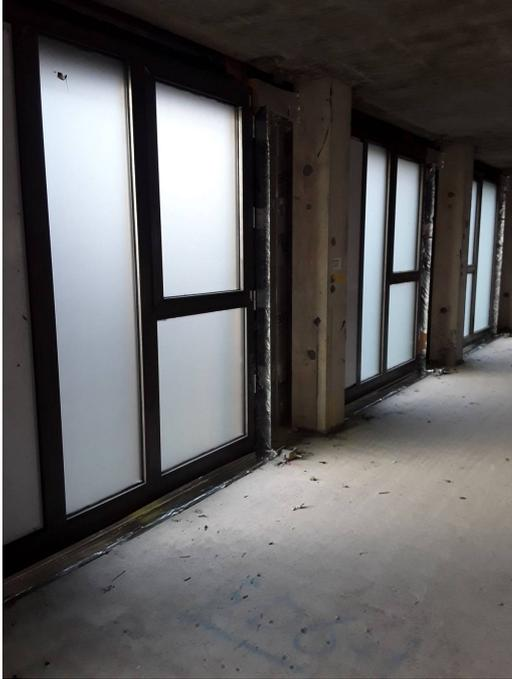
PeelGard® is a high-quality coating that effectively protects windows from damage during construction. When sprayed or rolled on, this protective solution forms a skin-tight plastic film over the window and frame, creating a barrier against damaging elements.
