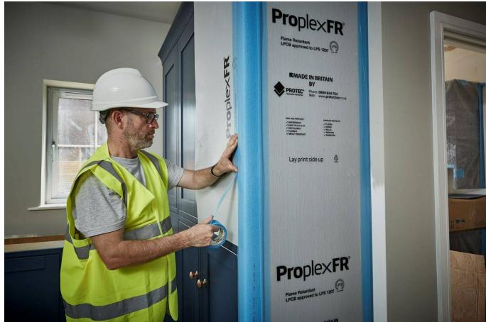
**Flame retardant (LPS 1207), twin wall, impact resistant sheets can be used to protect most finishes including floors, walls, doors, windows and workops. Available in several thicknesses and weights which can be selected based on site traffic and project duration.**
