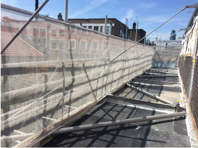
FR Vented Debris Netting can be quickly and easily fixed to scaffolding & Heras fencing for an FR debris solution.
