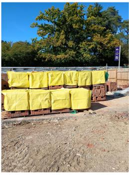
Brickshield Pallet Covers feature a UV coating to maintain their hi-vis yellow colour, protect against material deterioration, and enhance waterproofing. Two sides include extra 'wings' along the bottom edge, which can be weighted down to keep covers
