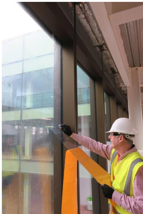
**ArmaSkin is a clear heavy duty and high performance temporary protection film for glass facades. With a unique adhesive coating, Armaskin is easily removed without leaving a residue. Can be in place for up to 12 months without replacement.**
