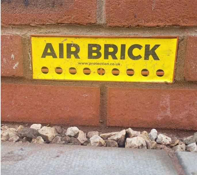
Adhesive covers to minimise debris passing through the air brick whilst allowing air to continue to circulate
